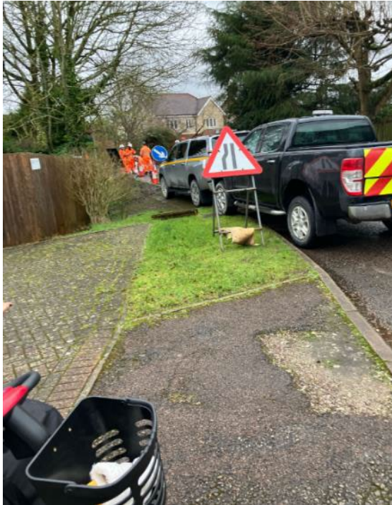
Figure 3 Contractors' Parking Blocking Bridleways, Feb 25 (note resident's wheelchair in foreground)
