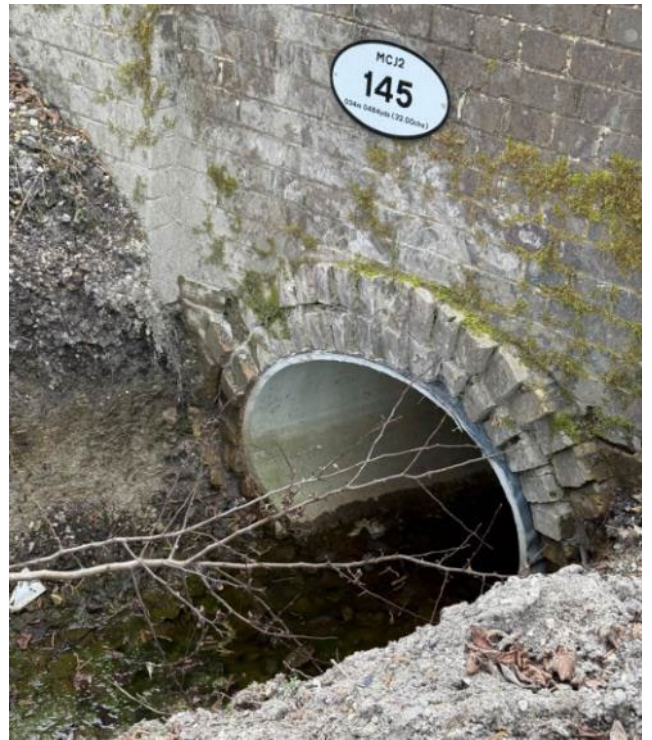
Figure 4 Network Rail Culvert MCJ2 145
